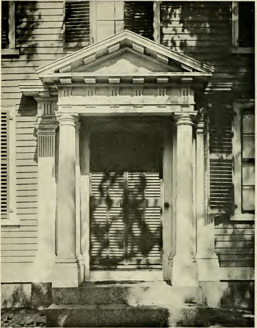
PLATE XIX.—Porch of the Stearns House.
